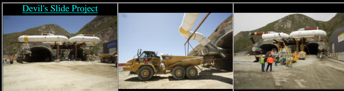
Highway 1 Devils Slide bypass project south of Pacifica, CA.
